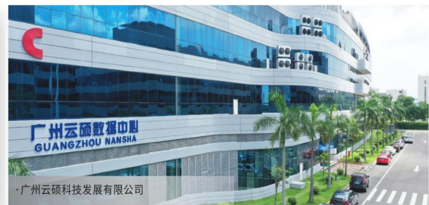
Build-to-suit multi-storey workshops
