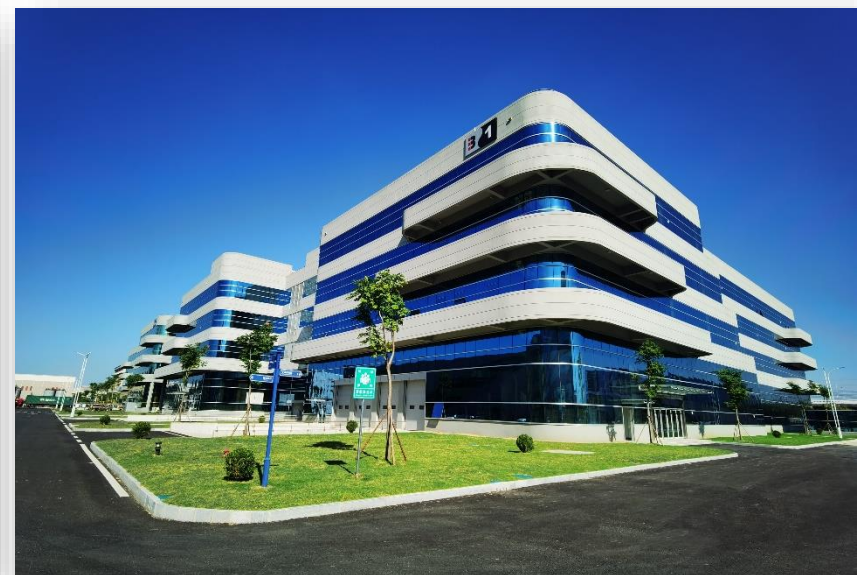
High-end multi-storey workshops
