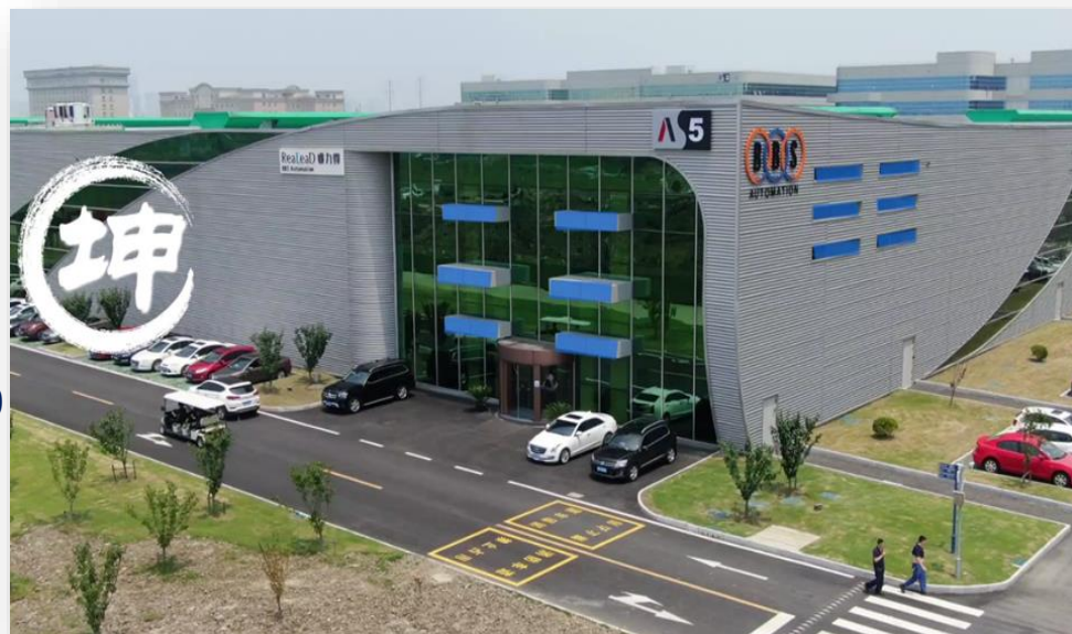
High-end single-storey workshops
